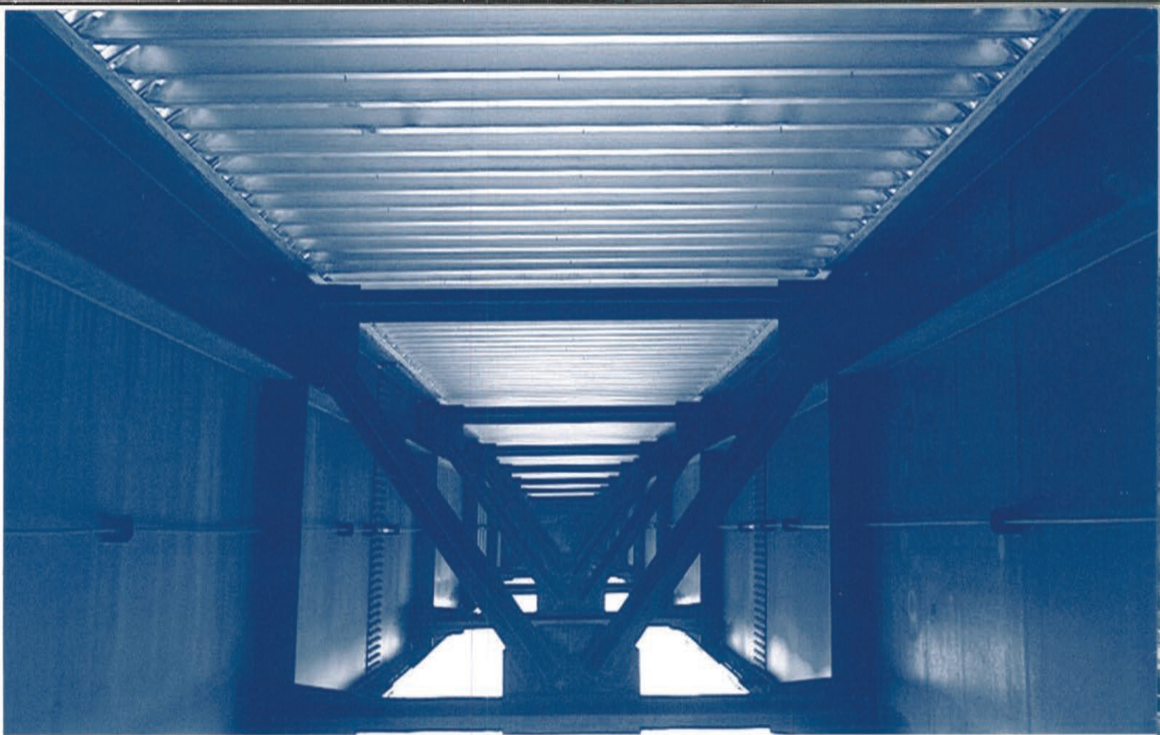
(Above) Bottom view. No forms to remove.
