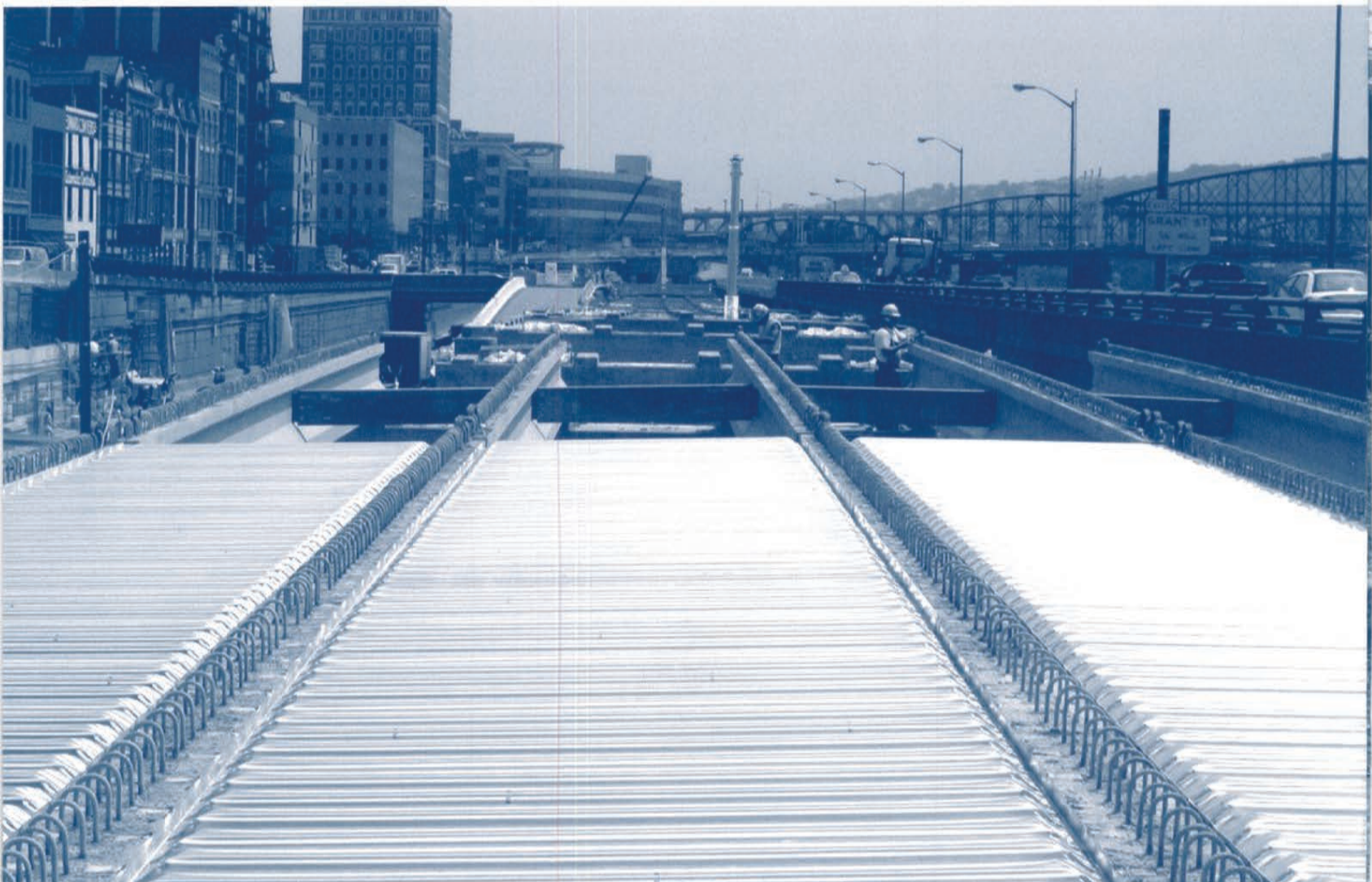
(Below) Top view of deck awaiting rebar and concrete
